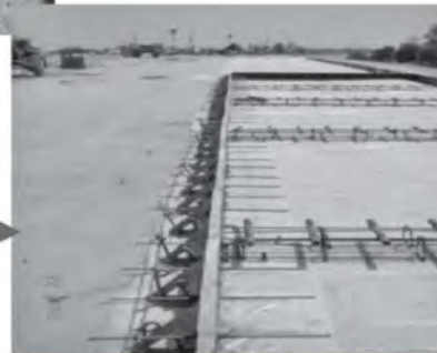
Properly aligned Tie Bars Placed in Side Form Holes
