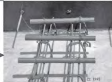
60% Dowel Length Covered With Plastic Sheathing and Dowel Chairs Designed Properly
