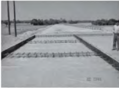
60% Dowel Length Covered With Plastic Sheathing and Dowel Chairs Designed Properly
